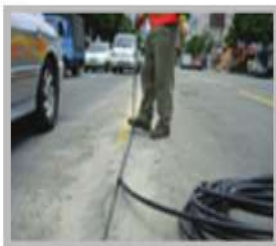
5. Bury the CD cable duct
