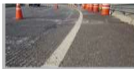
Installation of Lane at Roadside
