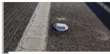
Installation of Shoulder Lane
