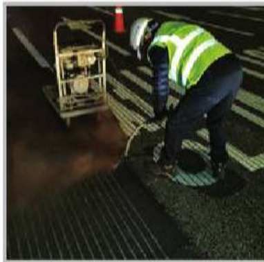
2. Clean with air after perforation
