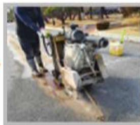
2. Cut the road
