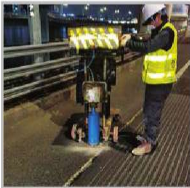
1. Perforation for Roadstud Installation
