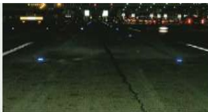
Entrance of Hi-Pass Section of Seohae Grand Bridge
