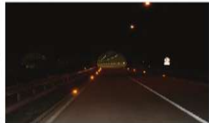
Entrance of Jangseog Tunnel of Honam Expressway
