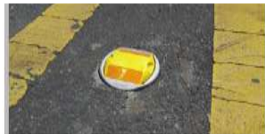
After Installation of Roadstud at Road Centerline
