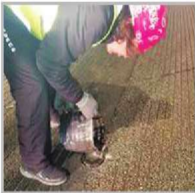
4. Put epoxy adhesive in perforation site
