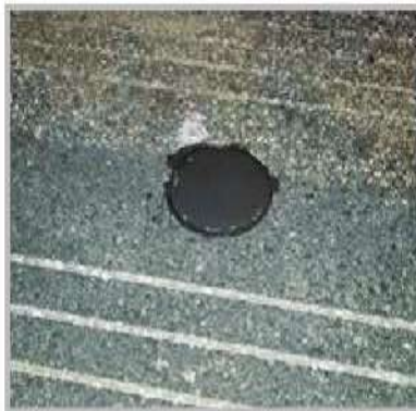
5. After putting epoxy adhesive
