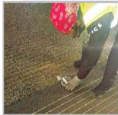
6. Inserting roadstud into the site
