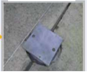
8. Install road reinforcement plate
