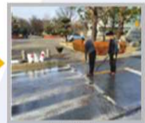
4. Clean the road
