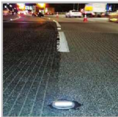
8. After installation of roadstud 2
