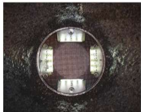
LED Roadstud that was installed 10 years ago
