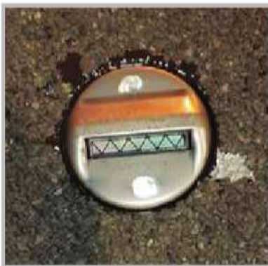
7. After Installation of roadstud 1
