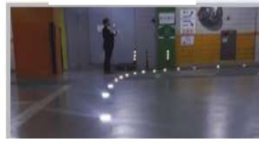
Installation of Indoor Parking Lot
