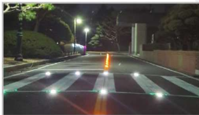
13. View after Installation
